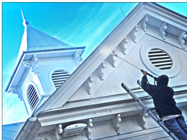
Fall Cleaning: worker power washes Carlin Hall as part of the building's ongoing preventative maintenance.
