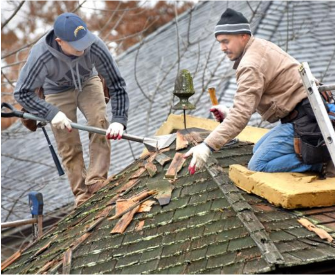
Workers from Kirby Kerns beginning the work of removing moss-covered and curling gazebo shingles in December 2019
