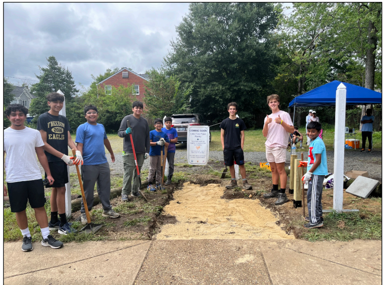
Boy Scout volunteers working on installing the pantry; photo credit Mohammad Dannan
