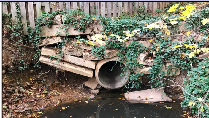
The damaged concrete pipe
